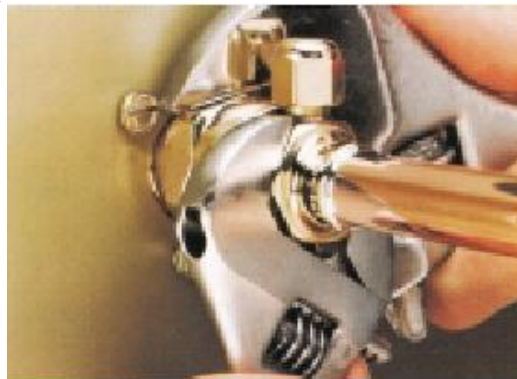
Tighten Swivel Nut
