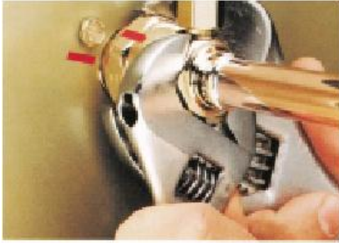
Rotate Swivel Nut ¼ Turn More
