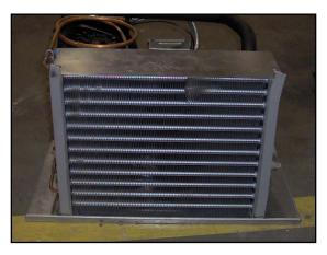
**Condensing Units:** Once a month compressed air should be blown through evaporator to clear any debris or dust – opposite to direct normal air flow.
