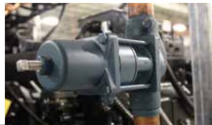
Figure 1-11. Condenser returning valve
