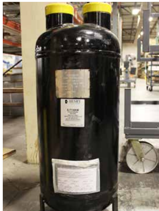
Figure 1-15. Suction accumulator
