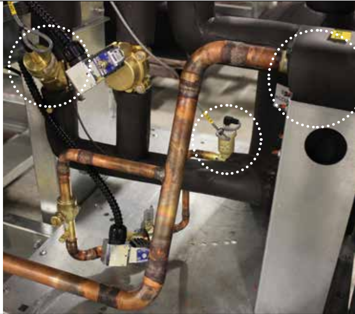
Figure 1-14. Subcooling assembly
