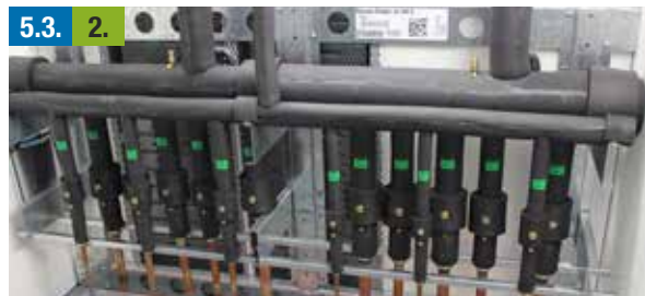
Figure 5-3. Refrigerant Charging
