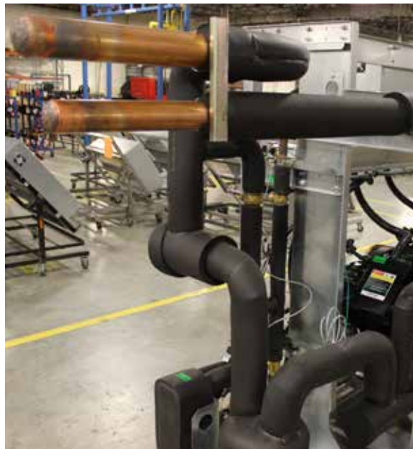
Figure 1-18. Example of the single pair of in a loop configuration leaving/returning to the rack (before being hooked up)
