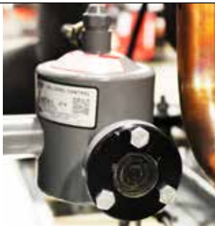
Figure 1-6. Oil level control
