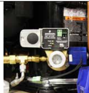
Figure 1-7. Compressor crankcase oil level protective control
