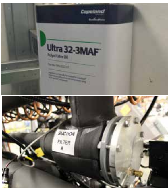
Figure 6-1. Examples of Compressor Oil and Suction Filter
