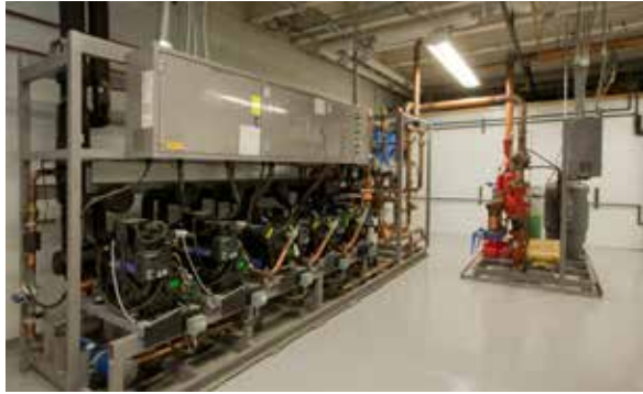
Figure 3-7. Rack Mounted on Floor
