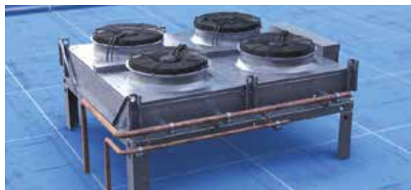
Figure 1-10. Air cooled condenser
