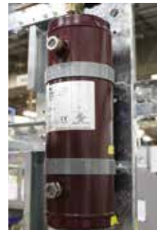
Figure 1-5. Centrifugal oil separators reservoirs
