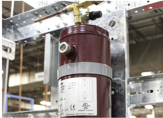
Figure 1-13. Oil reservoir
