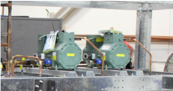
Figure 1-8. Low temrerature compressor (LT)
