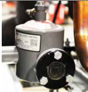
Figure 1-6. Oil level control
