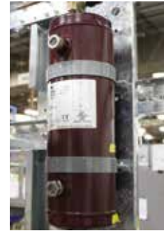
Figure 1-5. Centrifugal oil separators reservoirs
