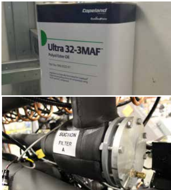
Figure 6-1. Examples of Compressor Oil and Suction Filter
