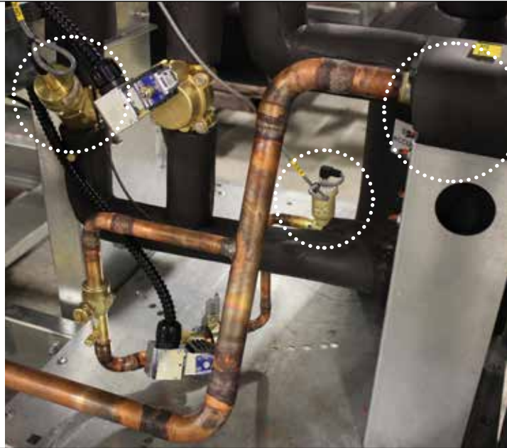
Figure 1-14. Subcooling assembly
