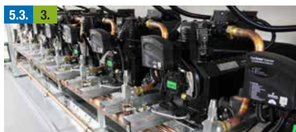
Figure 5-4. Starting Compressors
