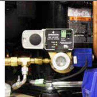
Figure 1-7. Compressor crankcase oil level protective control
