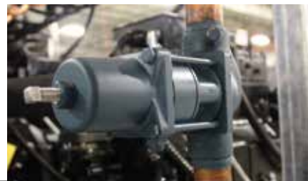
Figure 1-11. Condenser returning valve
