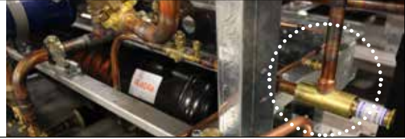
Figure 1-13. Liquid receiver pressure valve
