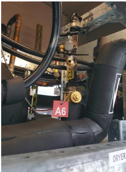
Parts are labeled to assist personnel in easily identifying and locating key parts of the system.
